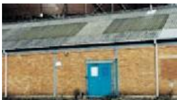
Corrugated roofing / cement sheeting
