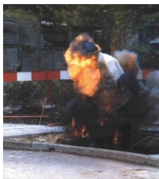
Photo of a HV cable damage incident Damage to services
